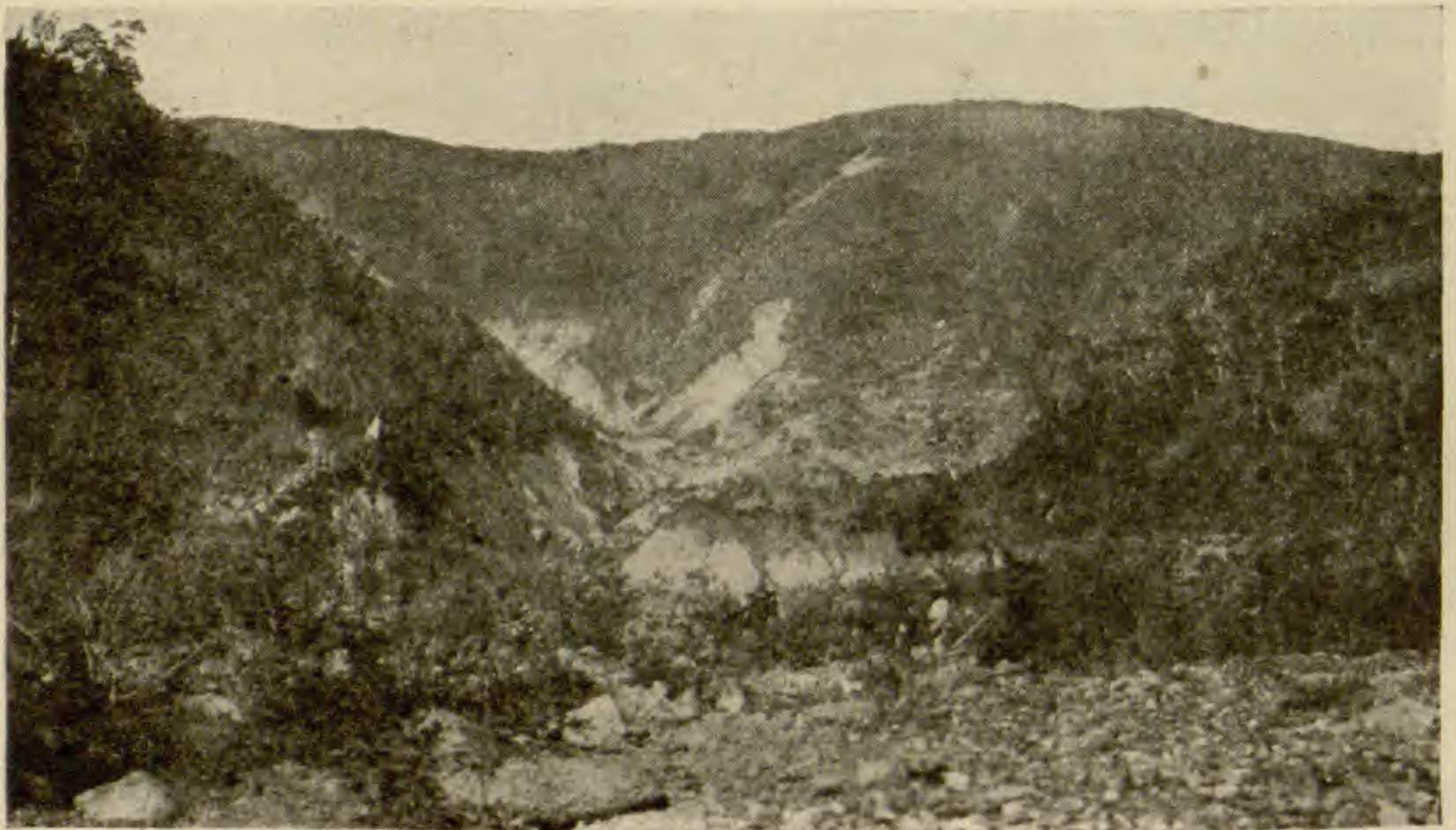
FIG. 2.—Looking north over upper Cascade Valley, showing scars left on south side of Blue Mountains by landslides.
